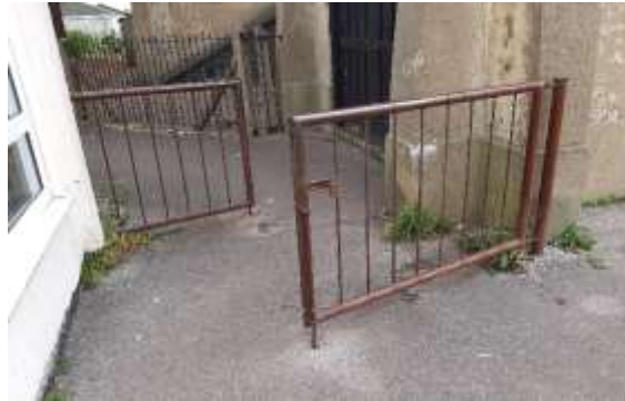
Figure 2 - Staggered barriers between the church hall (on the left) and the church (on the right).
